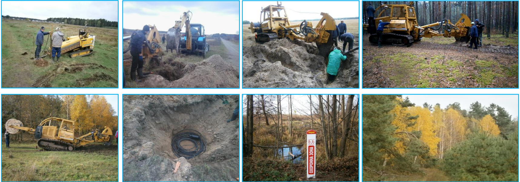
Fig. 4. The process of the fiber-optic communication lines installation.
