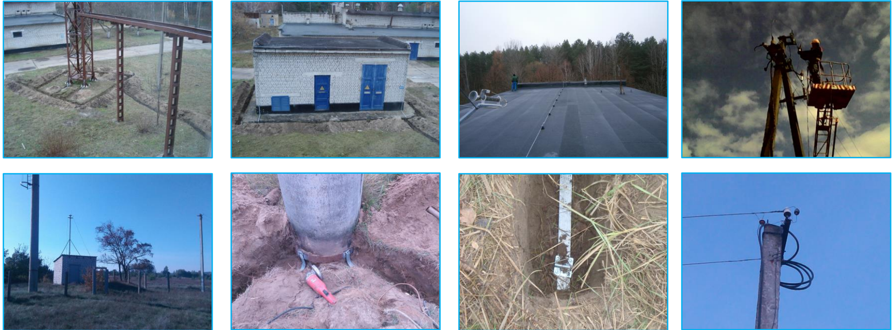
Fig. 3. The upgrade process of the grounding and the lightning protection system at the station sites.
