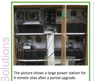
The picture shows a large power station for 4 remote sites after a partial upgrade. The upgrade was made without proper wires and materials available, leaving the installation messy and impossible to touch without high risk of damaging connections or equipment.
