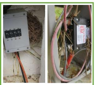
Circuit breaker box not installed properly because the right materials not available at the time of installation. Many of the wires used are not rated for the maximal current and lugs are missing. A rodent had build a nest in the box, creating a fire hazard. The box and wires were later replaced.
