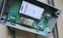
Two examples of flooded electrical enclosures showing fast corrosion due to electrolysis reaction, when the water reaches power terminals. The copper and other metals becomes electrodes that deteriorates very fast due to electron and ion-movement.
