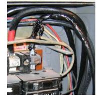
Examples of melted and corroded power wires due to poor electrical connections. The top picture shows a poorly connected wire from a photovoltaic panel which generated heat that melted the wire insulation and caused corrosion.
