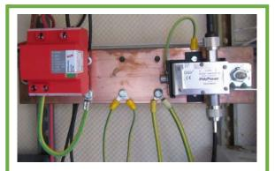
The picture shows a cleaned copper ground bar with new bolts and modern surge protection. Note the ground wire installed on the GPS surge protector in order to ensure a proper ground connection.
