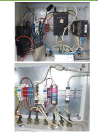
Power and communication enclosure before and after a maintenance upgrade. The installation was simplified due to advances and standardization of equipment, eliminating the need for port servers and a power converter. All status diodes are facing outward to the user for easier inspection and maintenance. The excess cables in the bottom of the enclosure were left mounted to avoid open holes.
