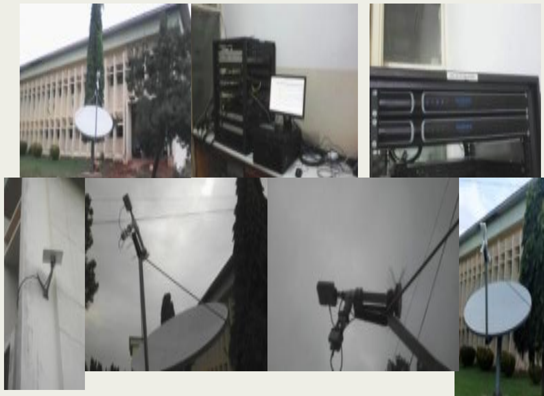
Installed (GCI-III) / VSAT equipment
