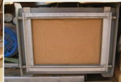
Filter clogged after just one day due to heavy dust
