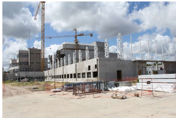
Northwest view of Neutron guide building. March 2022
