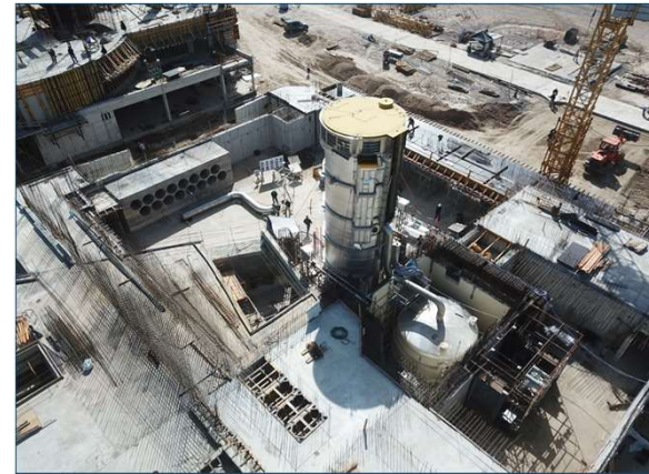
View of reactor pool – which is equivalent to the pressure vessel if it were a power reactor
