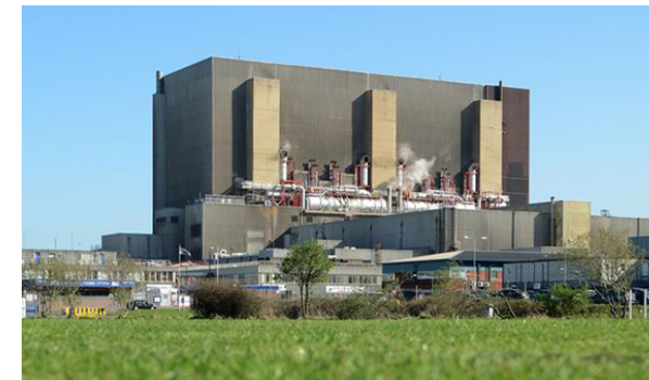
Hartlepool power station, located on the North-East coast of England
