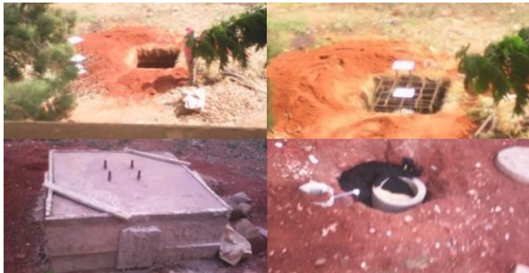
Fig. 1 Ground/concrete works for the (GCI-III) / VSAT equipment installation
