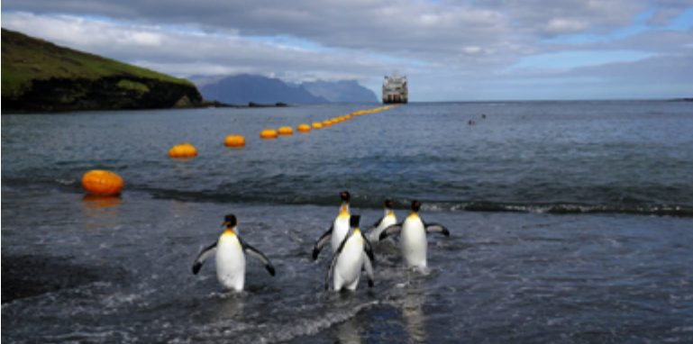
Figure 11. Trunk cable shore landing at the CTBT IMS hydroacoustic station HA04 (Crozet Island) utilizing improved vessel positioning and control systems. From J. Cummins et al. [T1.3-06].
